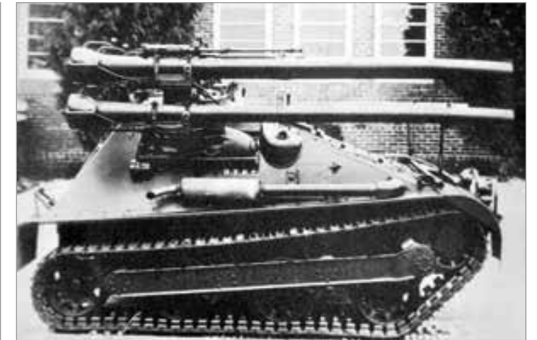
The impressive-looking M50 Ontos tank destroyer held a formidable rifle array which had to be reloaded from the outside of the vehicle.
